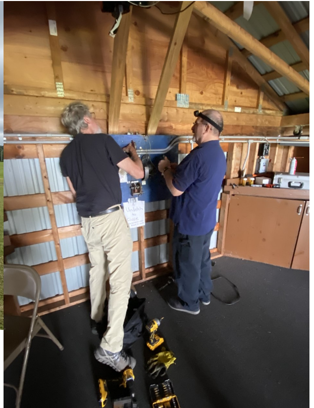
Jim and Dave doing maintenance on the cable pulleys.
