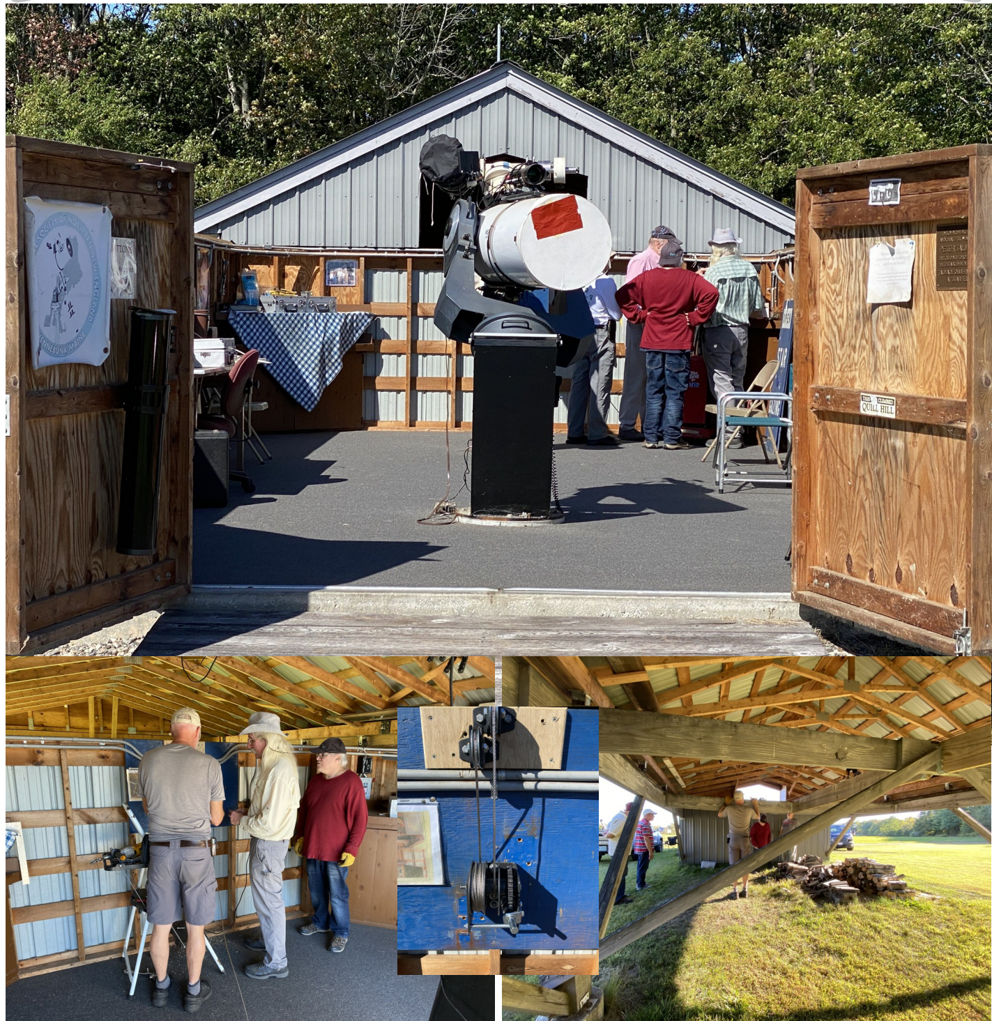
On Thursday & Friday the ASNNE crew installed a new pulley and cable system.
